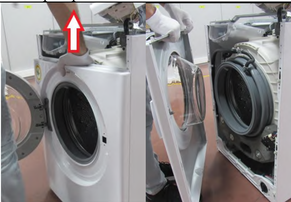
2.7.2 Pull up and remove the front panel.
