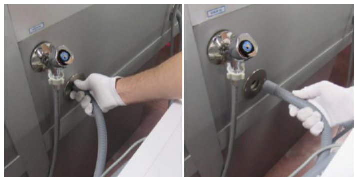
1.3 Disconnect the drain hose
