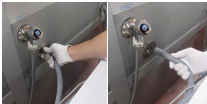
1.3 Disconnect the drain hose
