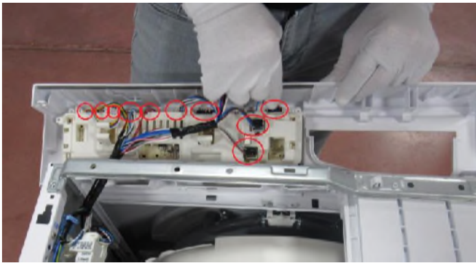
4.3 Connect the all sockets on the card according to the wiring diagram.
