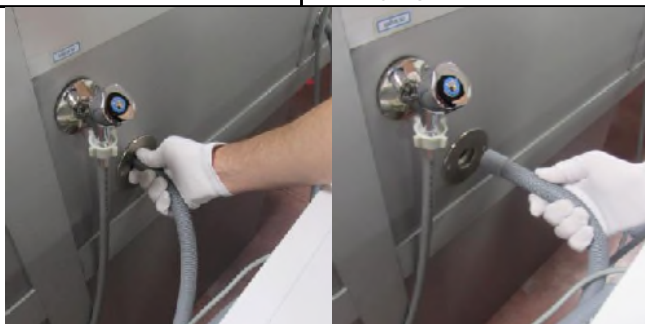
1.2. Turn off the tap and disconnect the hose from the valve
