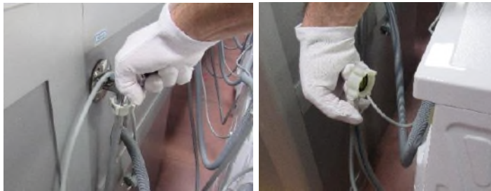
1.2 Turn off the tap and disconnect the hose from the valve
