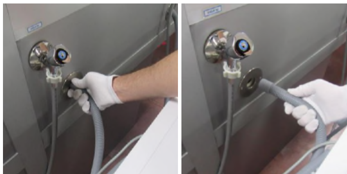
1.3 Disconnect the drain hose
