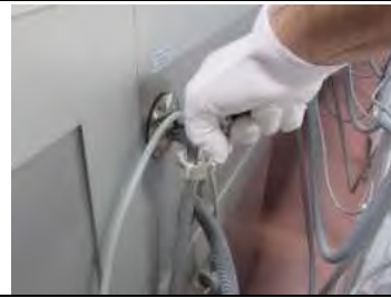
1.2 Turn off the tap and disconnect the hose from the valve
