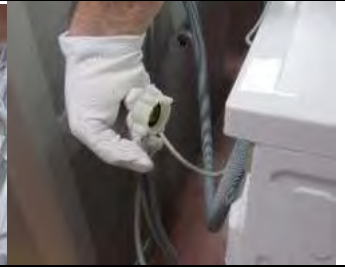
1.2 Turn off the tap and disconnect the hose from the valve
