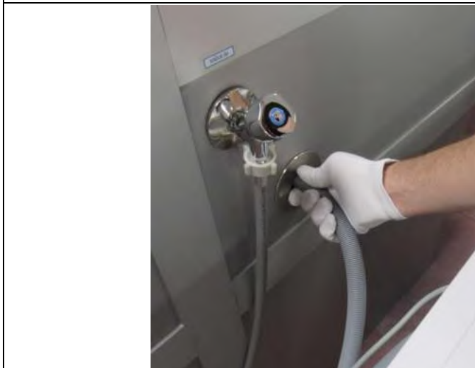
1.3. Disconnect the drain hose
