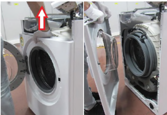
Pull up and remove the front panel.
