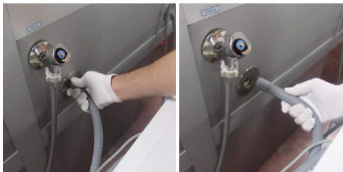
1.3 Disconnect the drain hose
