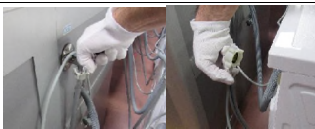
1.2. Turn off the tap and disconnect the hose from the valve
